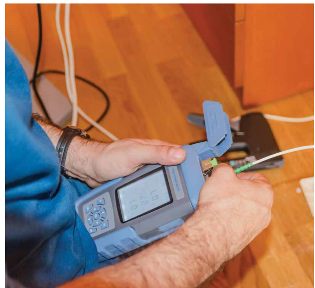
A technician measures the optical power loss after fiber installation.
