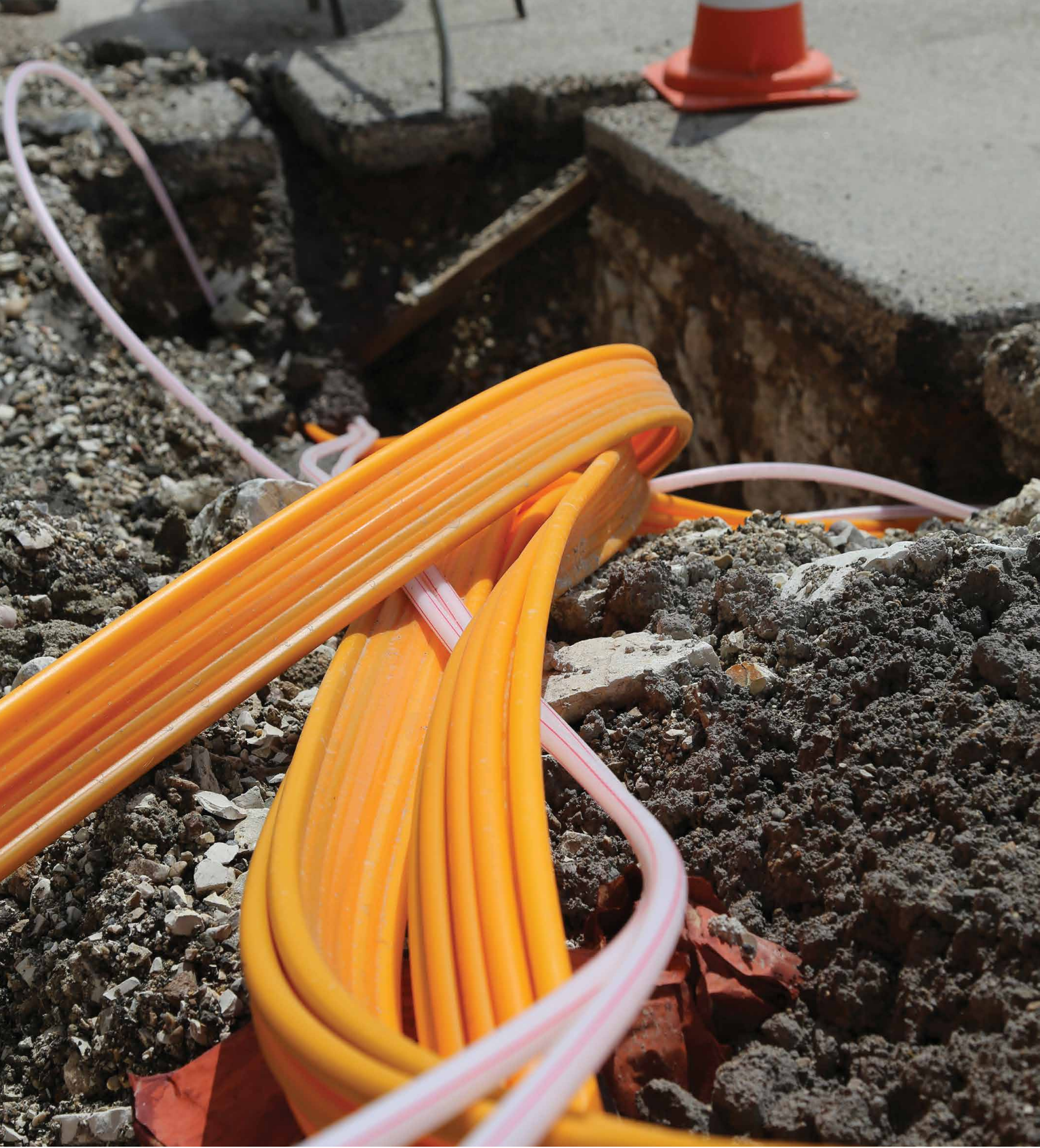
Road work for the installation of fiber optic cable.
